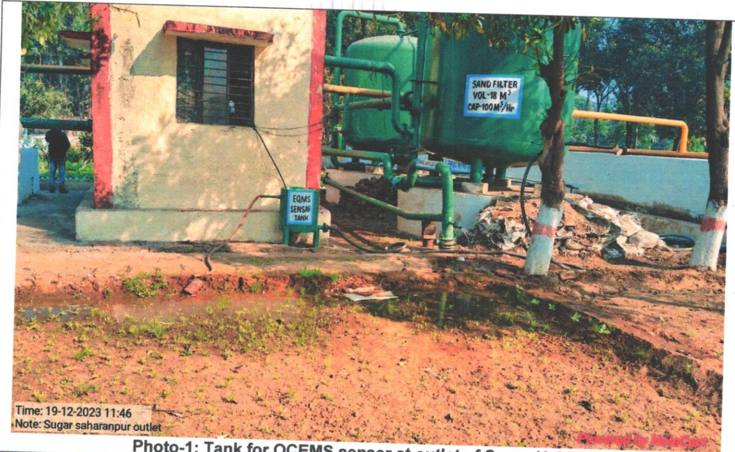
Photo-1: Tank for OCEMS sensor at outlet of Sugar Uni ETP
